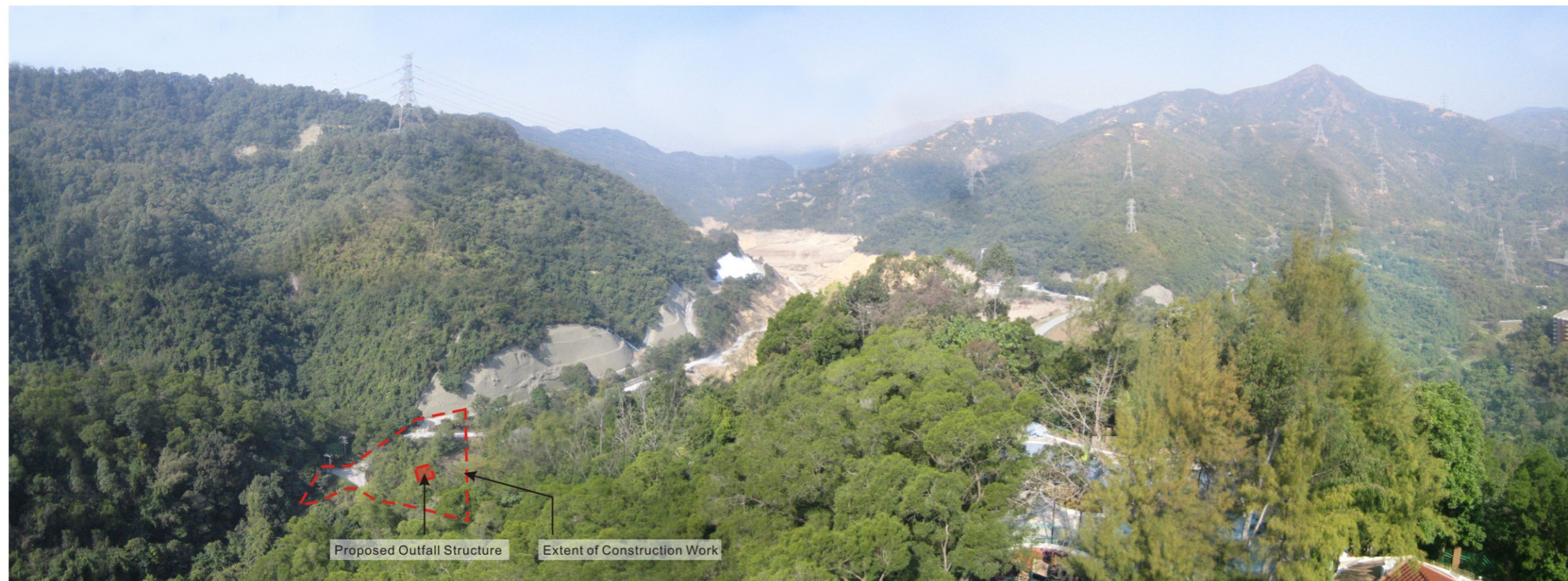
VSR R1 Residents of Lakeview Garden (Facing Northwest) (Following Construction)
