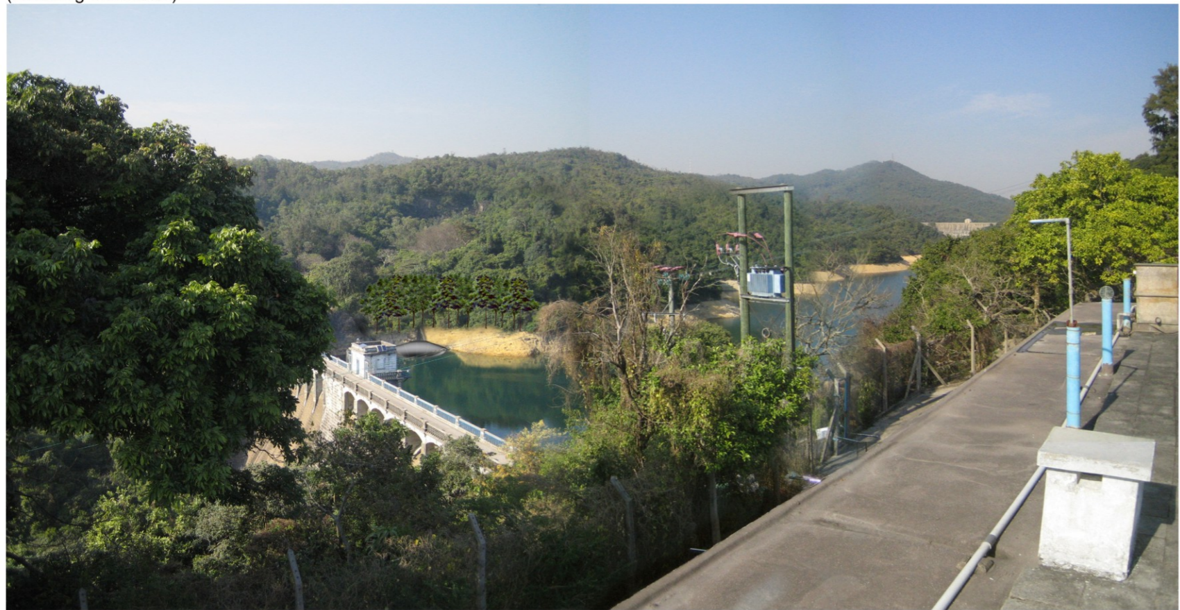
View from Abandoned WSD Staff Quarters (Following Construction)
